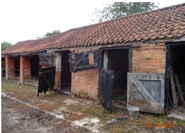
Site Photos Aug 2021
