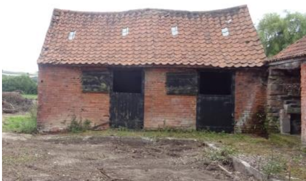
Site Photos Aug 2021
